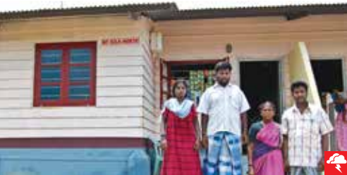
Duplex houses in Bamboo Flat, South Andaman
