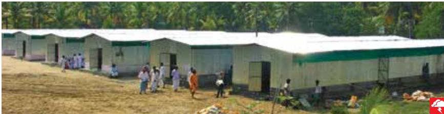
Temporary shelters in Kerala
