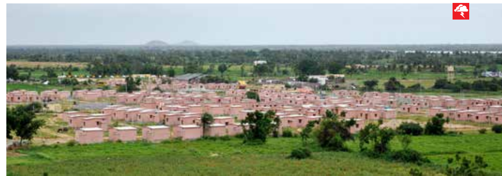
A view of homes built for displaced flood survivors in Raichur District, Karnataka
