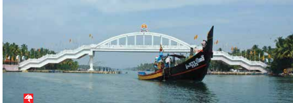
ETW's evacuation bridge, built over the backwaters of Kerala
